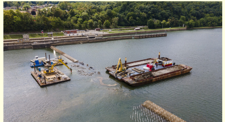
Contractors for the Pittsburgh Engineer District use floating barges to drill, demolish and remove rubble from the former Monongahela River Dam 3 in Elizabeth, Pa., on August 2, 2024, creating a 100-foot channel. (Photo by Michel Sauret/ Pittsburgh Engineer District)
