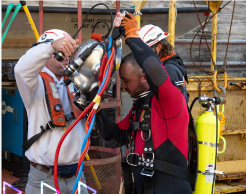
Ty Melton, a lock mechanic with the Corps' Nashville District, dons diving headgear with the help of Matt Williamson, a fellow mechanic at Wilson Lock, to dive-inspect the cracks in the land and river sides of the gates at Wilson Lock that closed on September 25. Photo credit: U.S. Army Corps of Engineers
