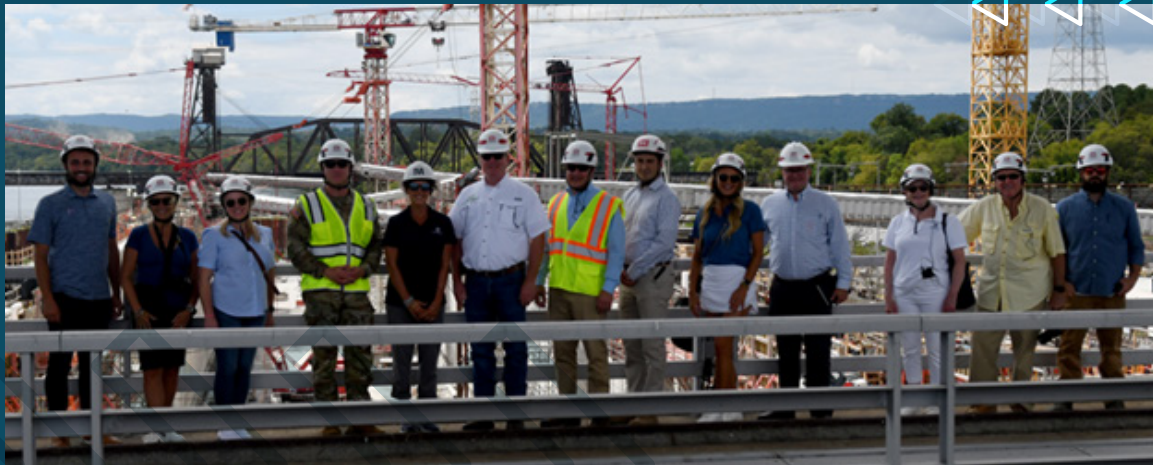
Participants of the 2024 WCI media tour stand at Chickamauga, as work continues on the lock replacement project slated to be operational in 2027.
