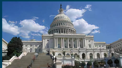
Attendees of the WCI February 7-9, 2023 meeting will visit with legislators on Capitol Hill to advocate for inland waterways priorities.
