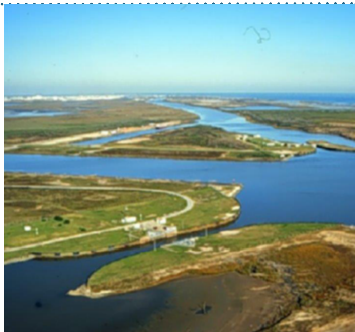
River Floodgates viewed from West to East.
