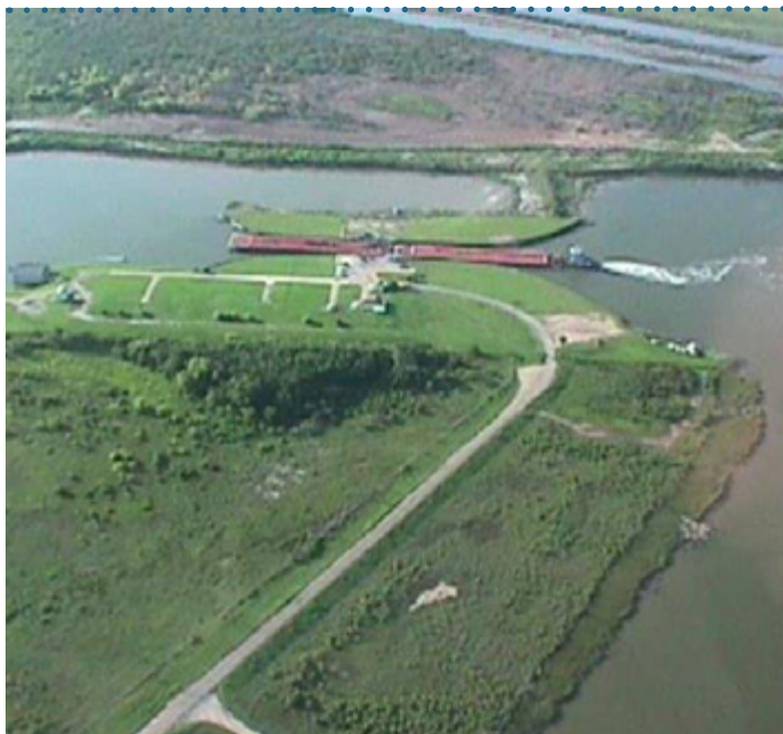
Current view of the East side of the Brazos River Floodgates.
