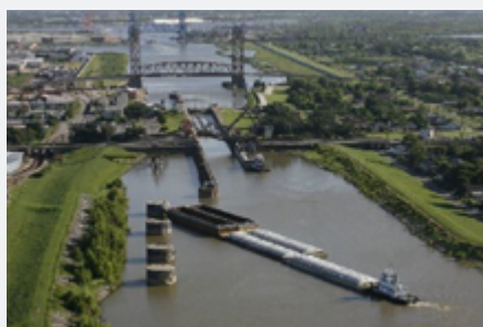
IHNC Lock is closed for 60 days to investigate leaking lock walls. Photo courtesy of GICA.
