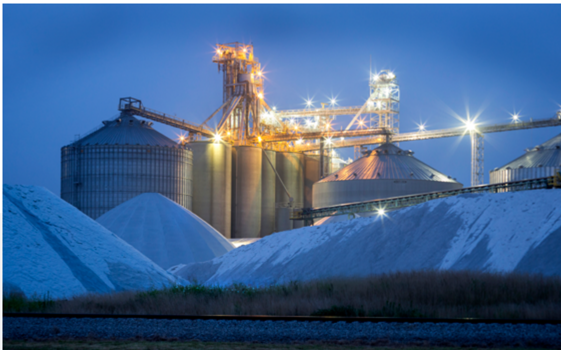
CGB's barge, rail and truck loading facility in Jeffersonville, IN.
