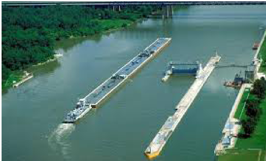
Peoria Lock and Dam in Creve Coeur, Illinois, will undergo dewatering for approximately 60 days for inspection and maintenance. Photo courtesy of U.S. Army Corps of Engineers.
