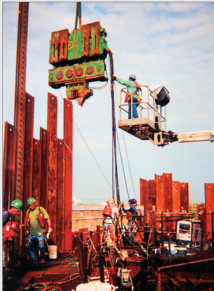
Above: A pile driver or vibro hammer is lowered by crane and placed on top of the steel in order to drive it into the riverbed, a job Richard Berry, of Metropolis knows all about as he was a pile driver foreman when he first began in 1993. He worked on the Olmsted project for a total of eight years.
