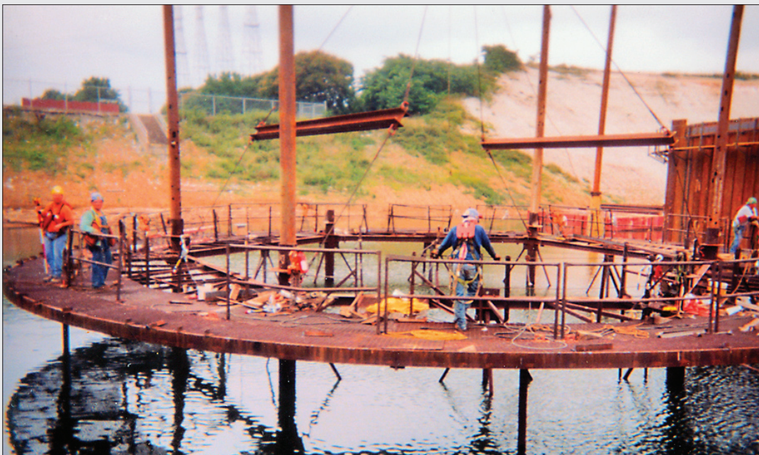
Above: The template construction workers used in 1993 to begin constructing the cells of the cofferdam.
