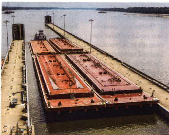
The towboat Stevn Holding , left, guides four empty tank barges through the Olmsted Locks in late July. The 1,200-foot chambers were completed in 2004 and have been used intermittently as construction continued on the dam. Below, five Tainter gates between the two locks and the wicket dam regulate the flow of water when all of the wickets are raised to fill the upstream pool.
