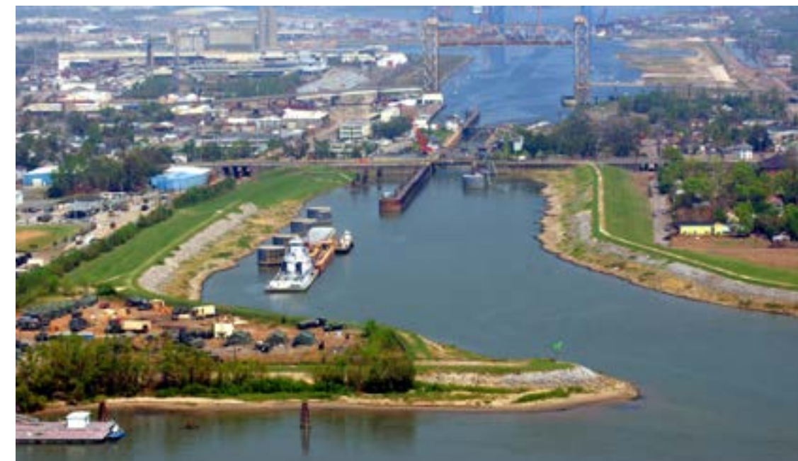
The Inner Harbor Navigation Canal Lock is located at the confluence of the Mississippi River and Gulf Intracoastal Waterway, the nation’s busiest and third busiest inland waterways.
